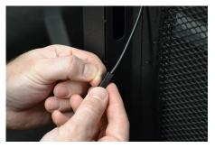
Peel the clear film from the adhesive on the sensor.
