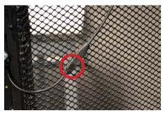
Connect the Sensor to the sensor cable on the RAC Lock body.
