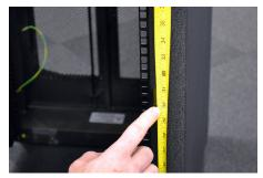
Mark the same position on the frame where the magnet will be placed.
