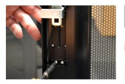
Align one of the brackets with the bottom screw inserts. Insert and tighten 2 of the screws to secure the bracket.
