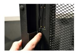
Remove the clear film on the adhesive and place the junction to hold the cable out of the way.
