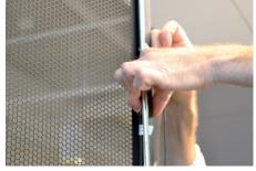
Route the cable up the inner channel on the door panel. Press the cable junction into the channel for at lest 10 seconds.
