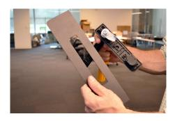
Remove the lock and the outer panel from the door. Set aside for later use.
