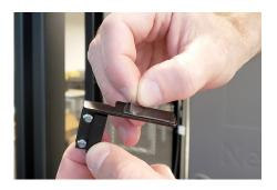
Peel the clear film from the sensor bracket at the end of the sensor cable.
