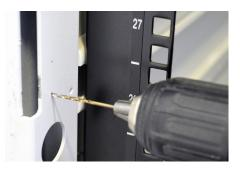
Drill the 2 pilot holes using a #44 drill bit.
