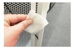
Use an alcohol wipe to clean the area that will align with the independent sensor installed on the opposite door.
