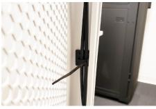
Loop the zip tie around the 2 cables. Trim the excess material.
