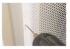
Drill 2 small pilot holes using a #44 drill bit.
