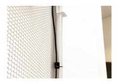
Place the cable manager in the cleaned area between the Rac Lock and the top of the door.
