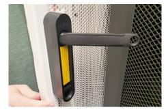
Turn the handle on the Rac Lock to the open position.
