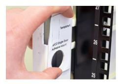
Place Template K onto the door frame so that the large hole in the template aligns with the hole on the frame.
