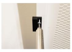
Align the holes on the sensor to the pilot holes. Secure the sensor to the frame using the included self tapping screws.
