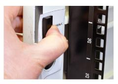
Place the sensor into the rectangular cutout in the template. Apply pressure for at least 10 seconds.
